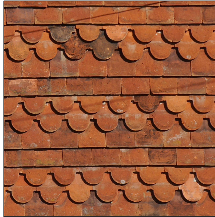
Tile hung wall [often with a mix of plain and scalloped tiles as above]
