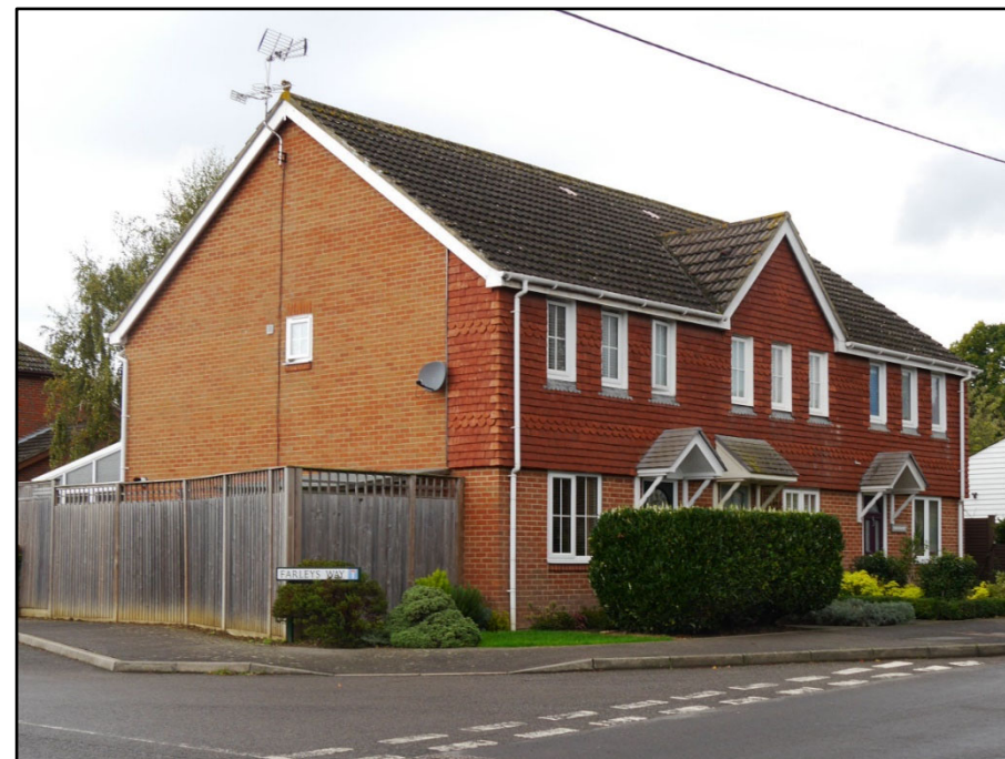
Some of the houses fronting on Main Street
