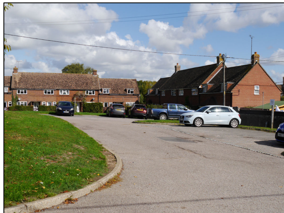
Houses in Park View, part of the 1960's or 70's Rother Estate, a mixture of 1.5 and 2 story dwellings
