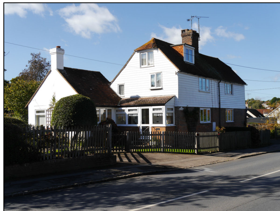
The Cedars / Spring Cottage, a pair of 2.5 story semi-detached houses lying close to the road
