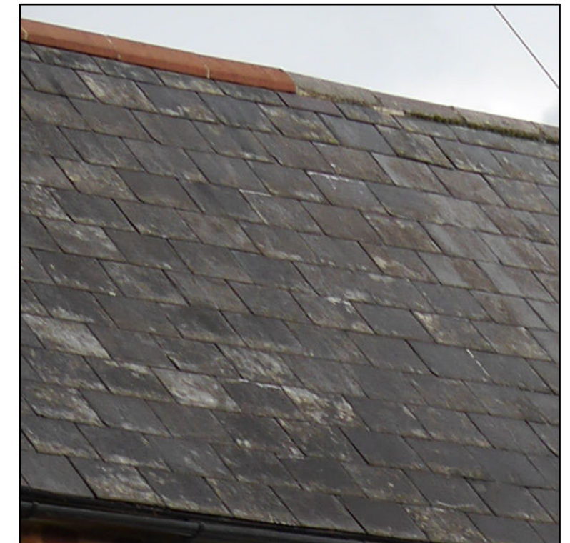
Less common slate tiles with clay ridge tiles can be seen in Peasmarsh
