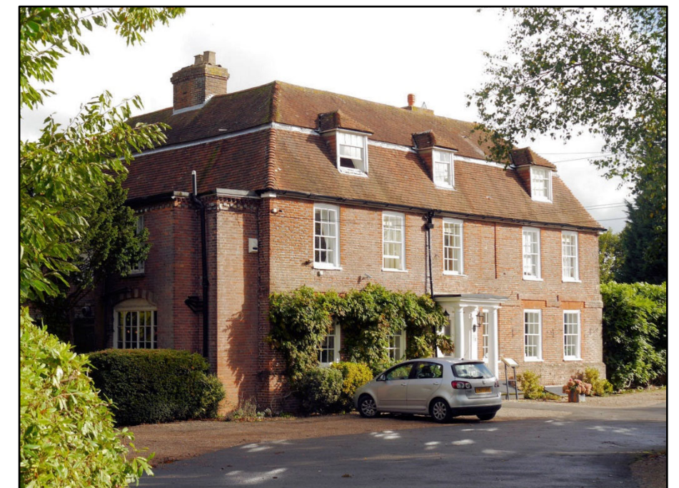
Georgian building at Flackley Ash Hotel
