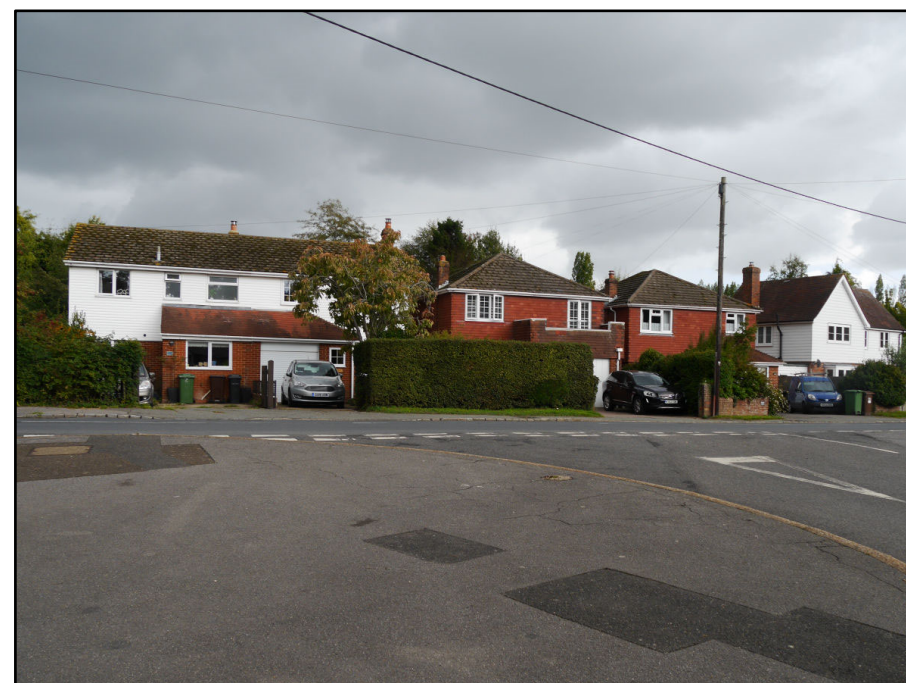
Modern housing on Main Street with tile-hung or weatherboard upper levels on brick lower stories
