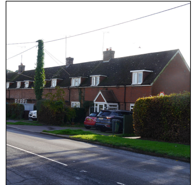
Separate, flat roofed dormers
