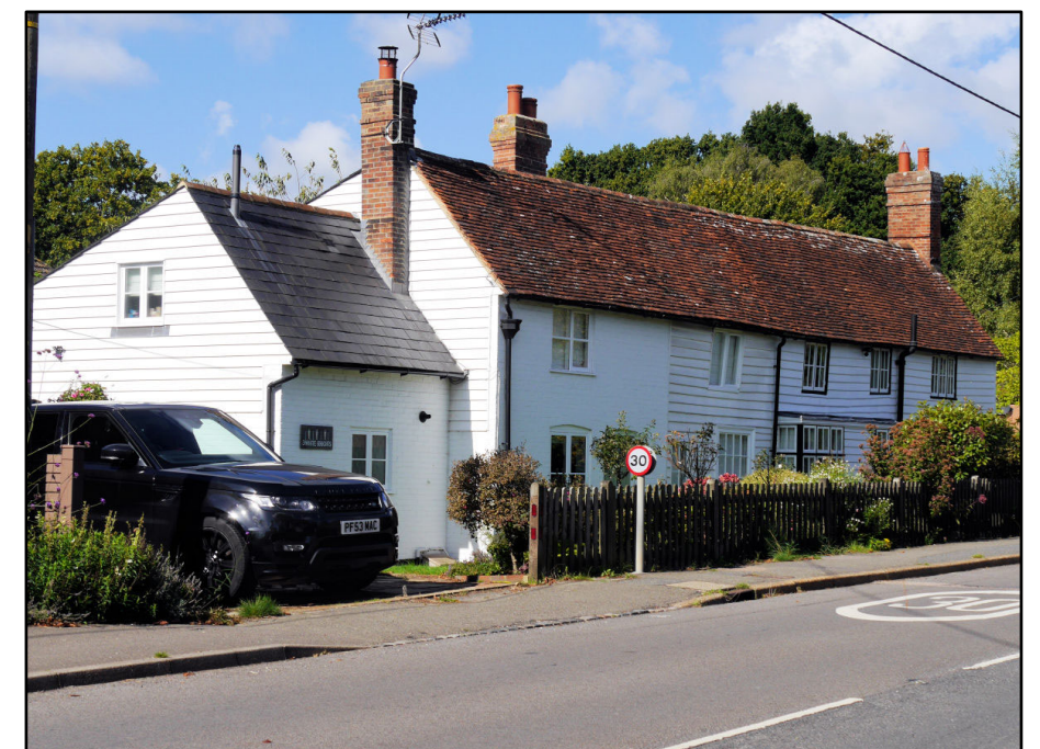
White Knights :Grade 2 listed semi-detached houses mainly weatherboarded but one section, presumably a rebuild, is painted brick
