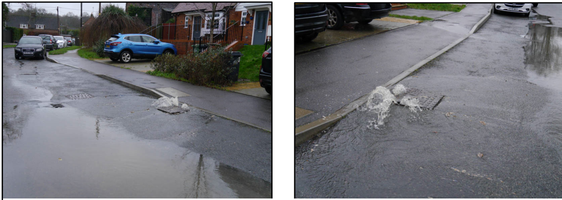
Major Foul Sewer Overflow 16/01/23 [SW Incident 4475539] [see also the short video taken just before daybreak]
